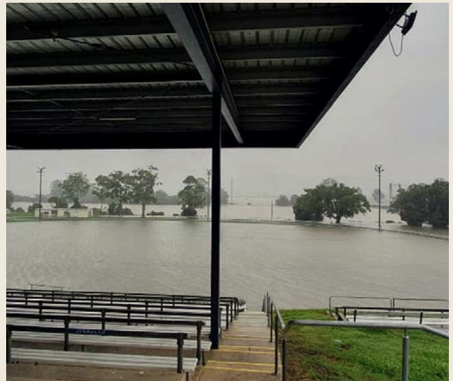
Figure 3.24 2022 Flood in Maclean Showground
