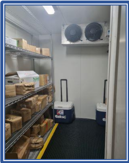
Event Freezer Refurbishment
