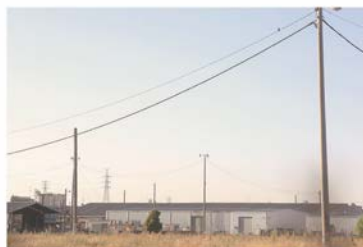
Above ground, power lines proliferate in a rhizome, commanding the landscape. Although highly considered, they arise with a perceived spontaneity, they impose themselves and grow tall, a series of connected monoliths.
