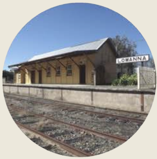
LOWANNA RAILWAY STATION
