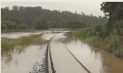
Freight train 4BM4 derailed due to a track washaway caused by heavy rainfall near Nana Glen in New South Wales.
