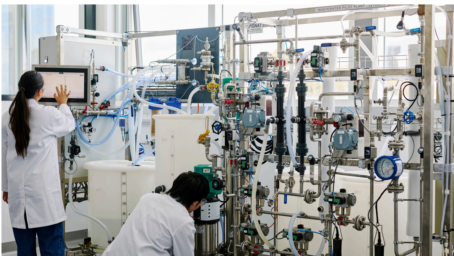
UF/RO Pilot Plant
