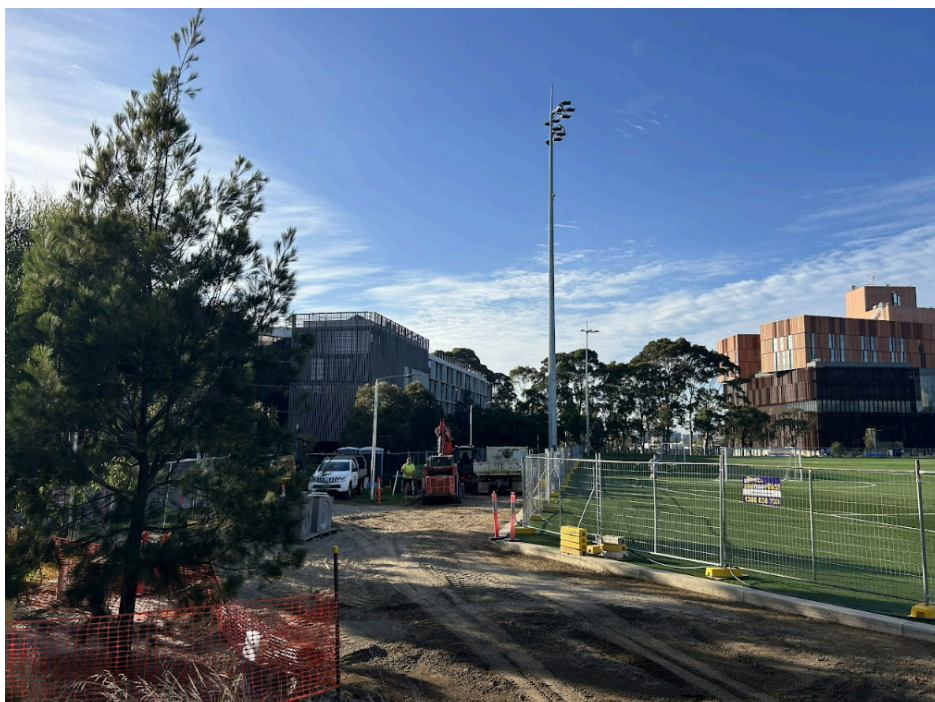
Image: The Tan Track is a ~1000m running track that encompasses Monash Sport's soccer pitches and football oval. Over the last few years, the University has made a concerted effort to gradually upgrade the Tan Track from compacted sand to sealed rubber composite. In 2025, the design documentation to seal the final section of the track was completed such that construction can begin in 2026
