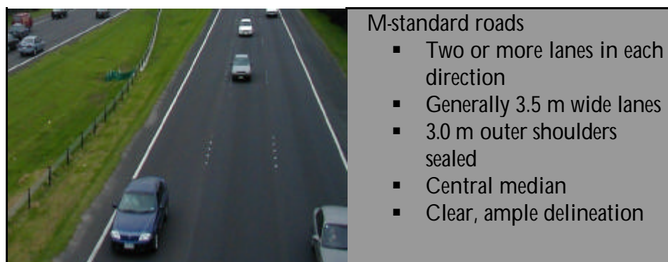
Typical Examples of Roads: Hume Highway and Monash Freeway
