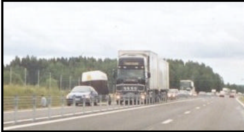
Figure 9 - Flexible barriers on site
