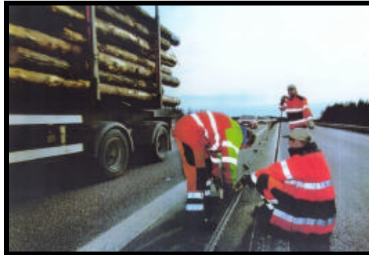
Figure 8 - Maintenance of barriers
