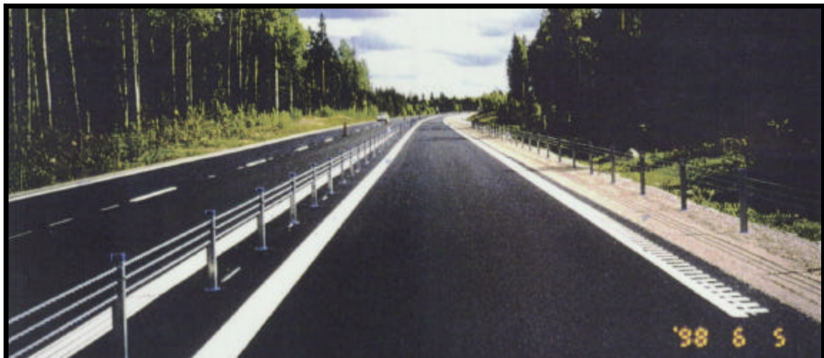
Figure 7 - Example of side and median cable barrier fence in a forest
