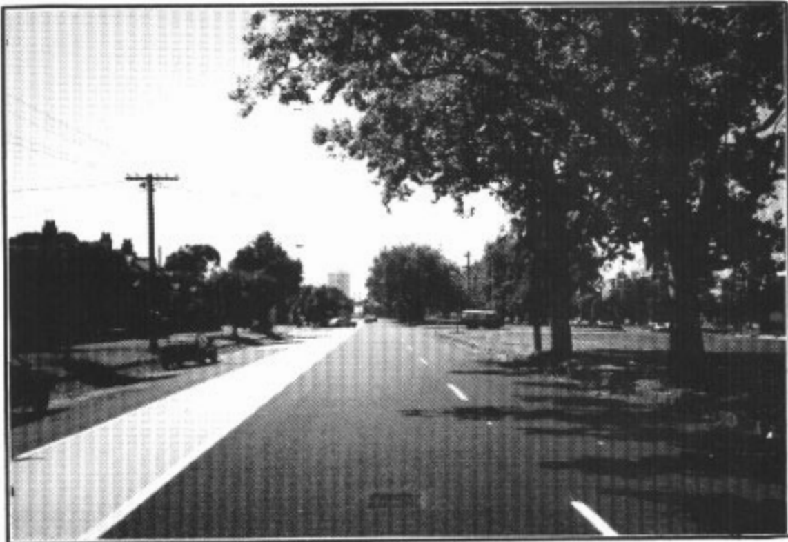
FIGURE 7.8 — Median and edge treatment on Lakeside Drive, Albert Park.
