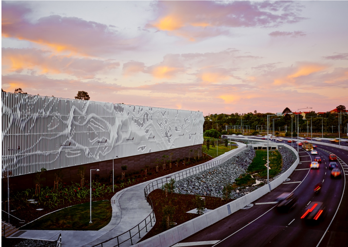
Figure 1. Legacy Way building façade manufactured by UAP. Photo Credit: UAP Company.
