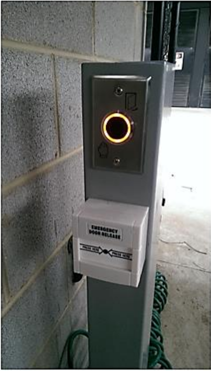
Fig. 1. Door release button and emergency door release. Please note that the gate must be kept open while using the facility.
