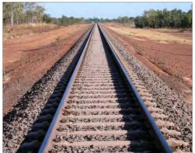
Railway Track with Concrete Sleepers
