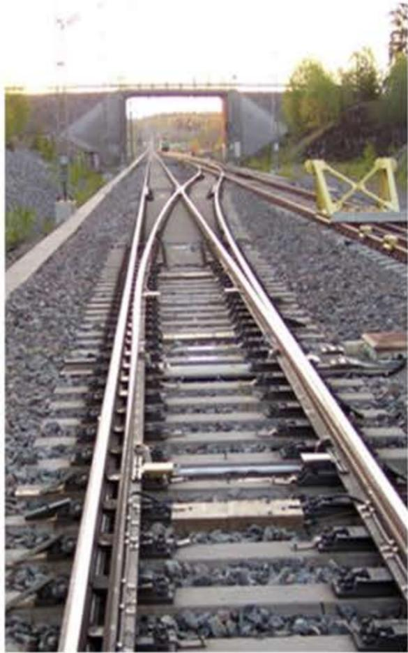
Dynamic train-track interaction in turnouts is far more complex than on ordinary tangent or curved tracks. The geometrical design, dictated by the function of a railway turnout, leads to additional disturbances compared to the normal response of a vehicle on plain line track. The largest disturbances occur when the wheels are transferred from stock rail to the switch rail in the switch panel and in the crossing panel when the wheels pass the gap between wing rail and nose rail.
