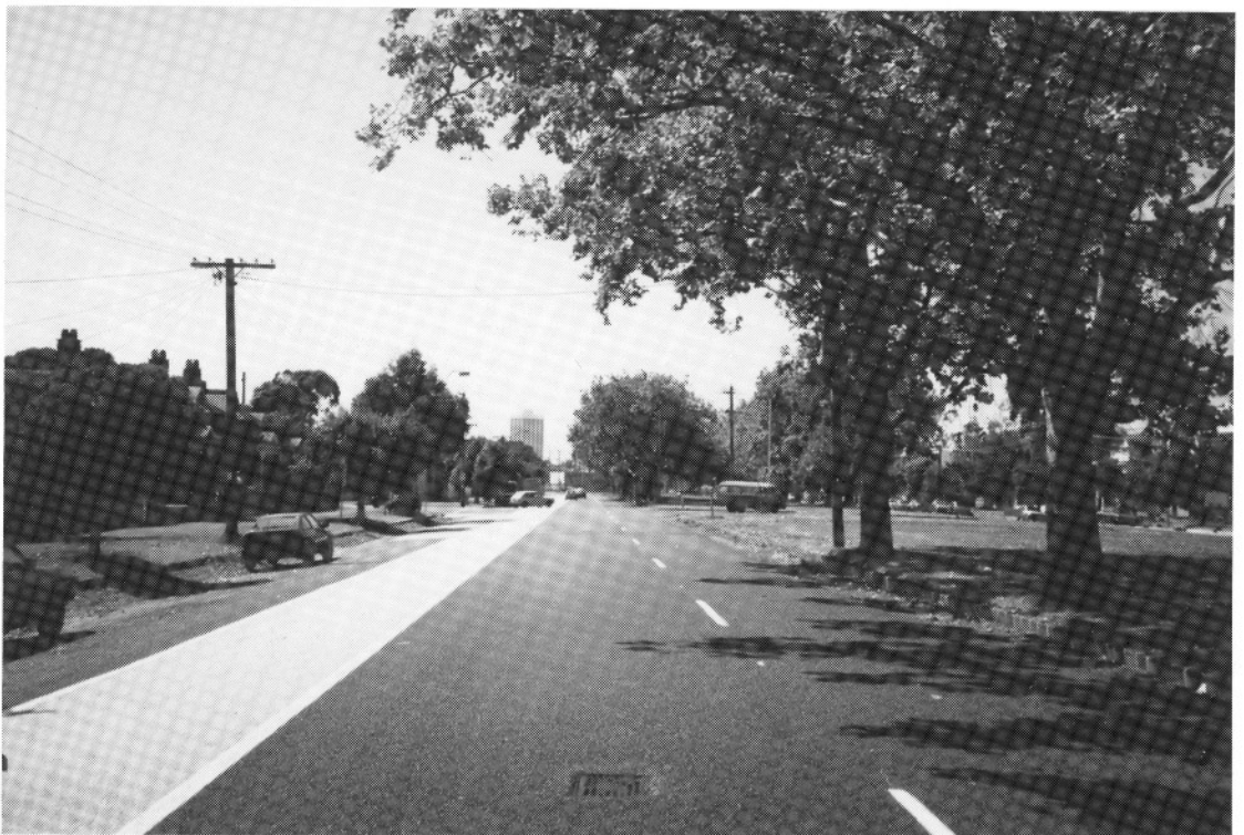
Figure 2.11 Perceptual narrowing treatment applied to Kerford Road, South Melbourne (from Fildes et al, 1989).
