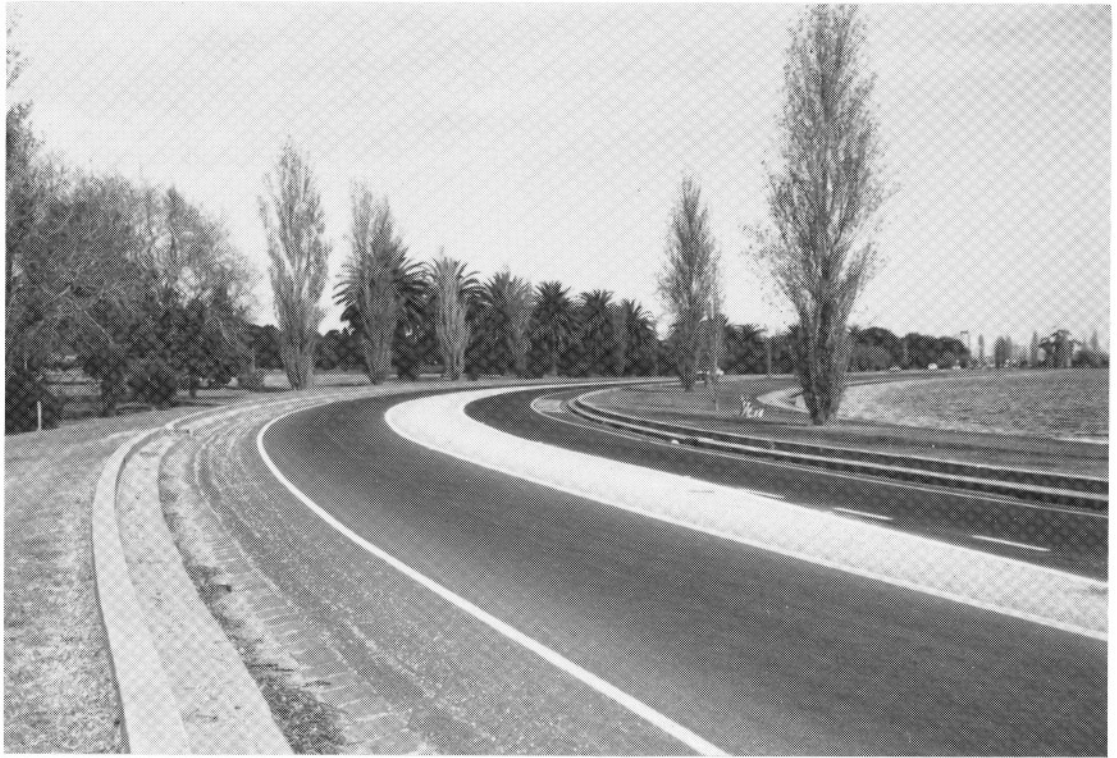
Figure 2.10 Median & edge treatment used on Lakeside Drive, Albert Park, Melbourne (from Fildes et al 1989)
