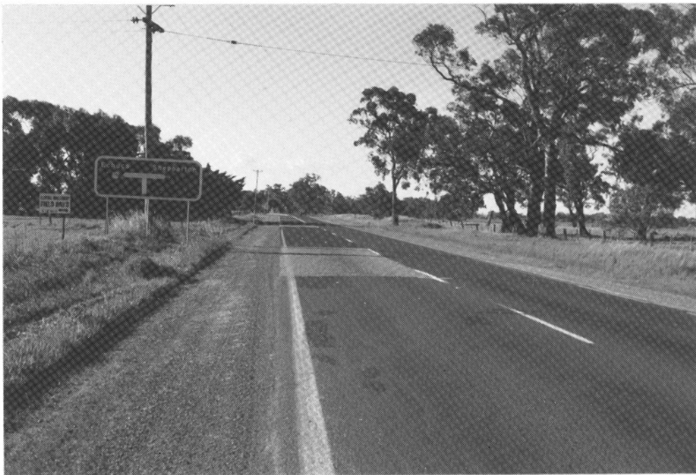
Figure 2.2 Transverse lines using different road metal on Northern Highway in Victoria (from Fildes, Leening & Corrigan 1989).
