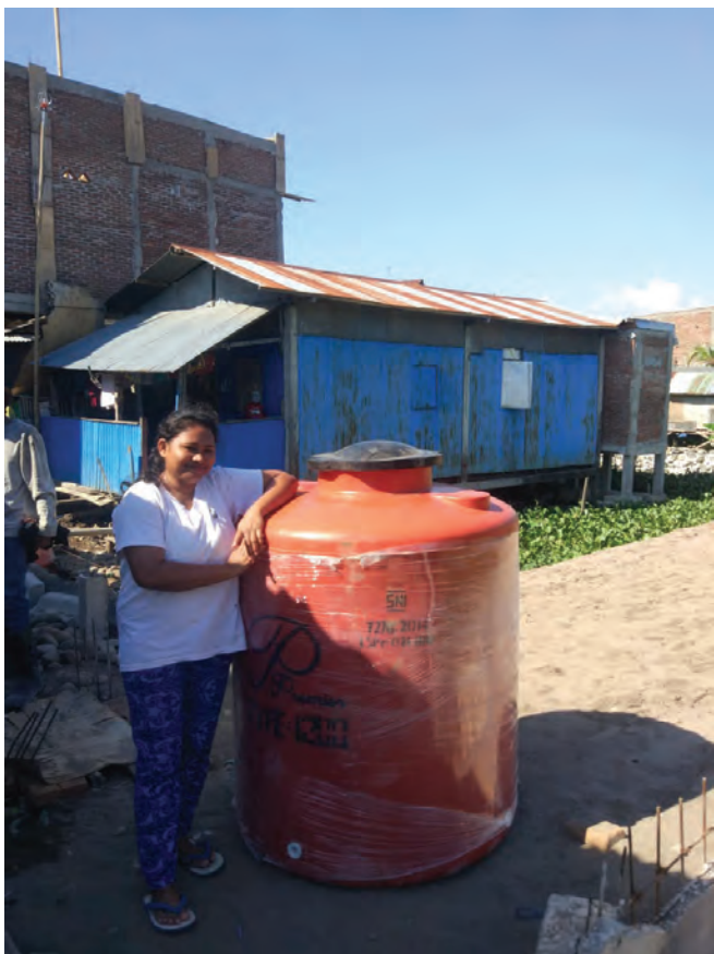
Rainwater tanks can provide buffer storage, reduce stormwater runoff, and increase water security, to complement reticulated supply.
