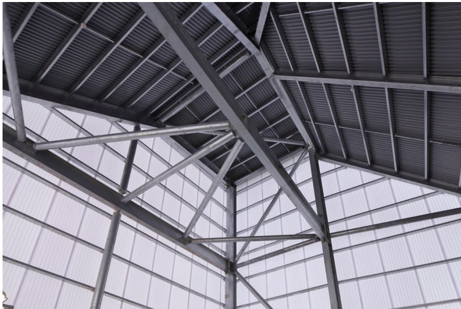
Figure 12. Exposed structure of the entry tower.
