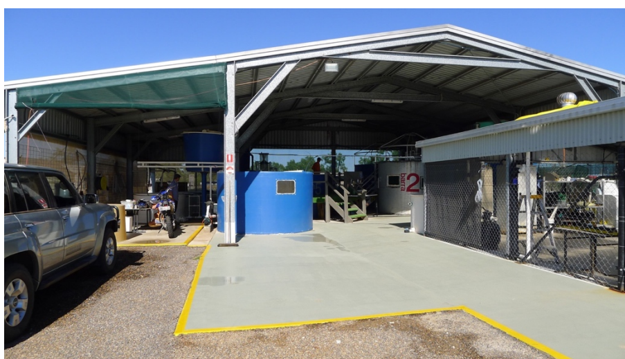
Figure 6. The existing Barramundi hatchery facility.
