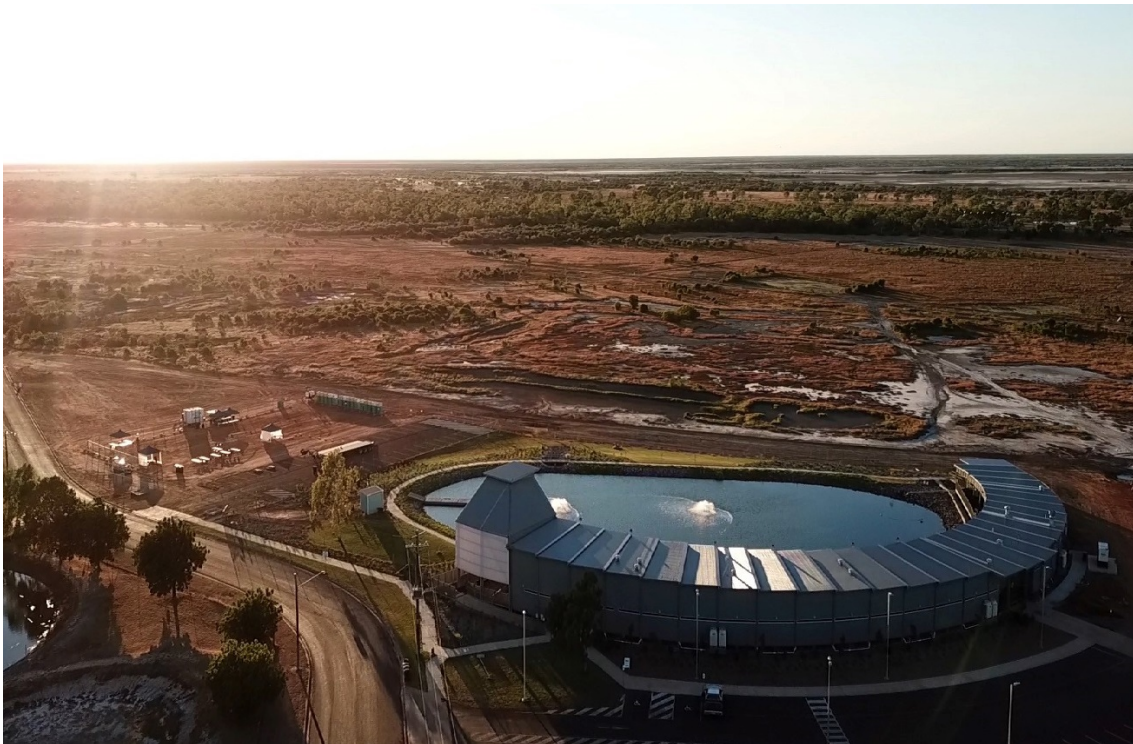
Figure 19. Drone footage of the completed LWBDC looking east towards the outback. 23
