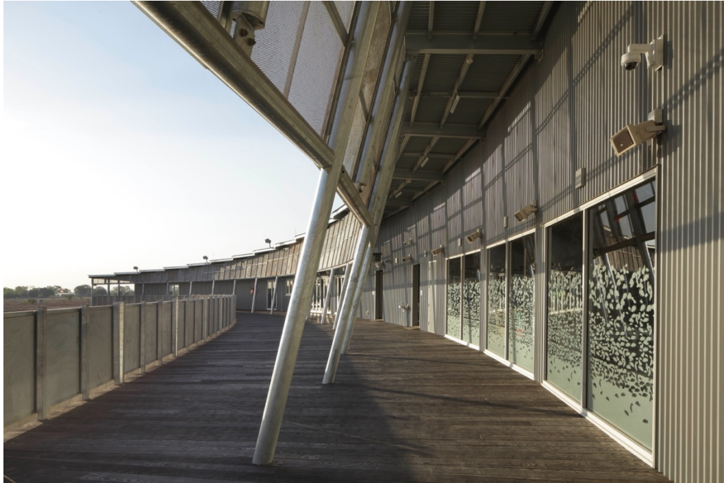
Figure 15. The curving verandah with angled columns and perforated steel screening. 18
