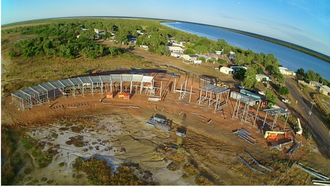
Figure 17. Construction progress monitored by drone. 20
