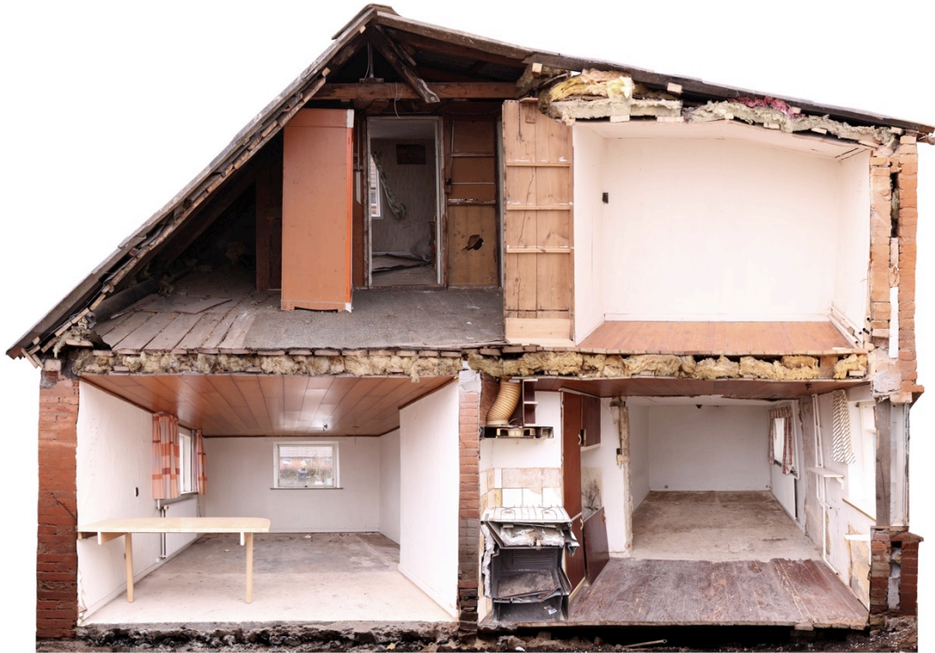
Figure 2. Section collage revealing the built chronology of a 150y townhouse (photograph by author).
