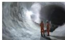
Sprayed Concrete Solutions for Tunnelling Projects
