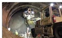
Lifting and Installations
