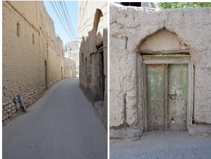
Figure 3 & 4. Traditional Omani mud settlement, common street view (left) & common entrance (Right). The Old Capital, Nizwa, Oman
