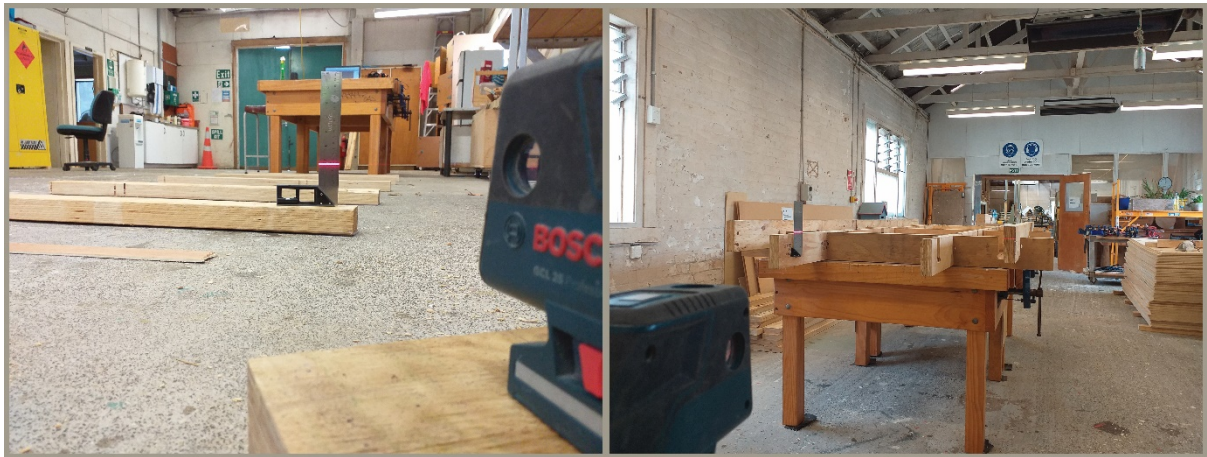
Using laser level and 0.5mm malthoid tape to 'pack' support elements.
