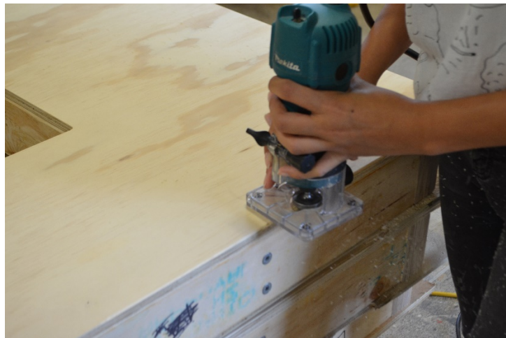
Edge Chamfering of Plywood to alleviate plywood issues – resulted in unique design feature.
