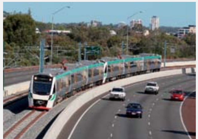
Figure 16. The first train on the Mandurah railway line.
