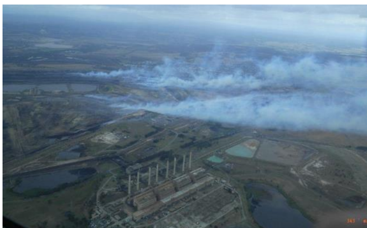
The Hazelwood mine fire, February 2014 Photo courtesy of Keith Pakenham, CFA Victoria
