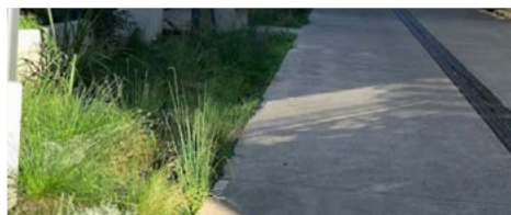
Kerbless road edges with garden beds for passive drainage
