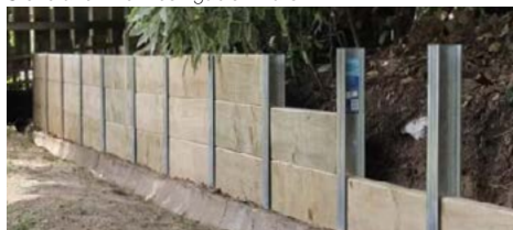
Timber and galvanised steel retaining walls
