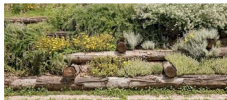
Log retaining structure
