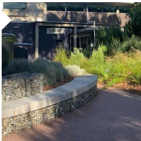
Stone and wire mesh gabion walls
