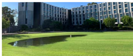
Detention basin w/ subterranean rain water tanks
