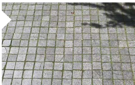
Hybrid Primary Walk paving, Ancora Imparo Way, CL
