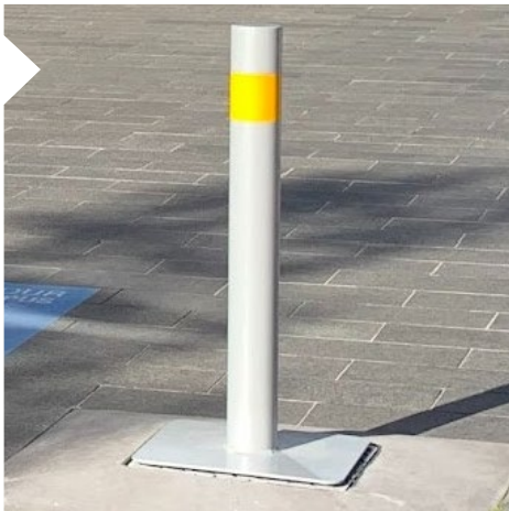
Bollard placed over malfunctioning retractable bollard
