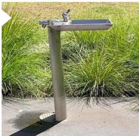
Drinking fountain w/ integrated drain installed in concrete
