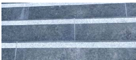
High contrast stone on stone stair nosing
