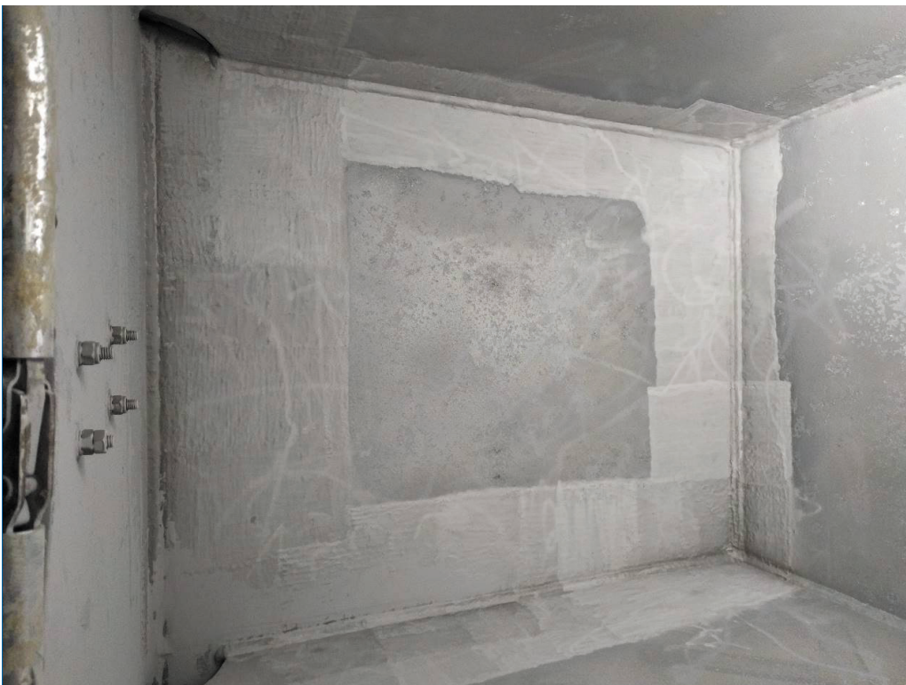
Deployment of cold spray as a coating repair technique for offshore structures. Read more about this project in pages 18 and 24.
