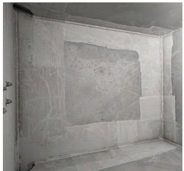
Crane boom tip box section showing the original TSA (darker grey) repaired with CSA (lighter grey), demonstrating the application of cold spray aluminium as an in-situ coating repair technique for offshore structures.
