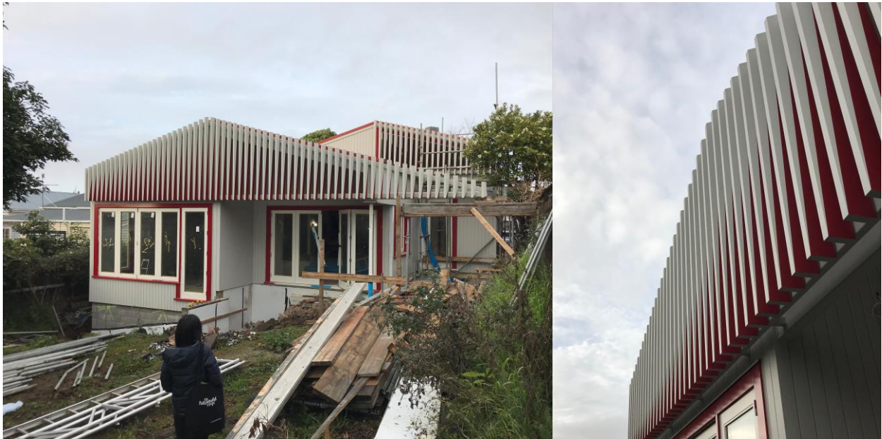
Figure 5. Paice Avenue splay cut timber screen under construction.
