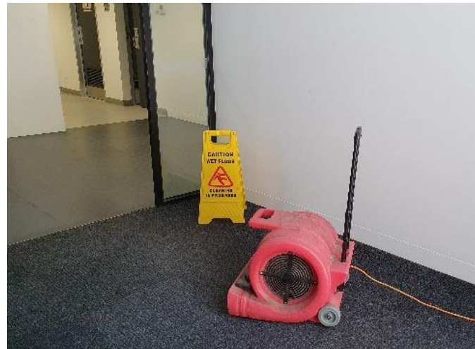
FIGURE 1: Example drying machine & safety signage
