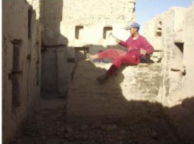
III. 31 Removal of dividing wall between rooms 5 & 6 on second floor
