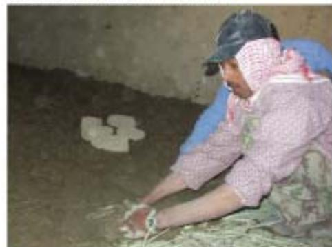
III. 30 Floor covering with mud and broken bricks
