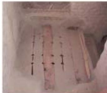
Ill. 22 Restored wooden floor with ventilation gaps in stairwell
