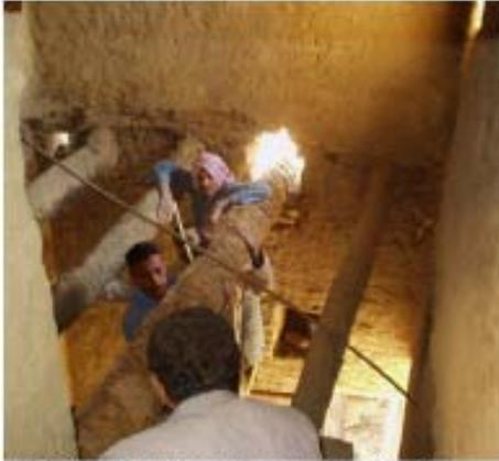
III. 24 New floor beam in room 3 on first floor
