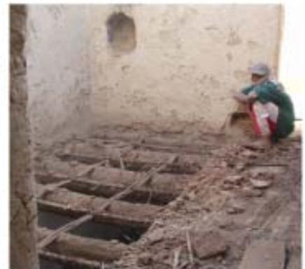
Ill. 23 Removal of damaged floor in room 3 on second floor
