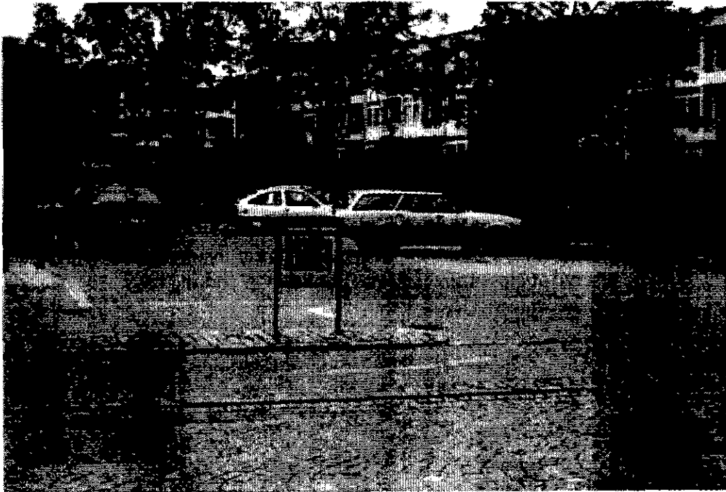
Photo 14: Herlev. (Local road (near library), 15 km/h advisory speed limit) Note: Pedestrian priority area. Distinctive pavement treatment. Parking allowed in area. Substantial trees and bushes.
