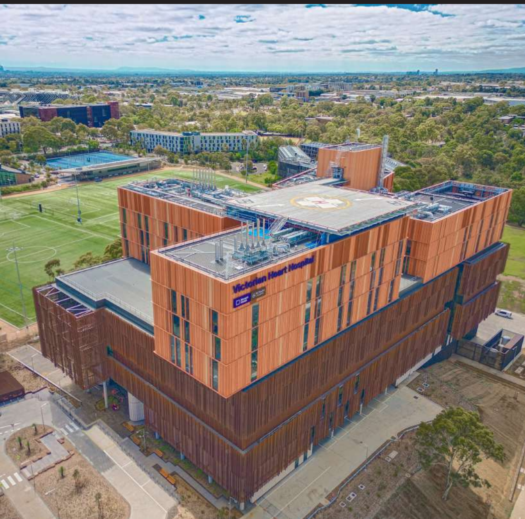
Victorian Heart Hospital – The first dedicated cardiac hospital in Australia.
