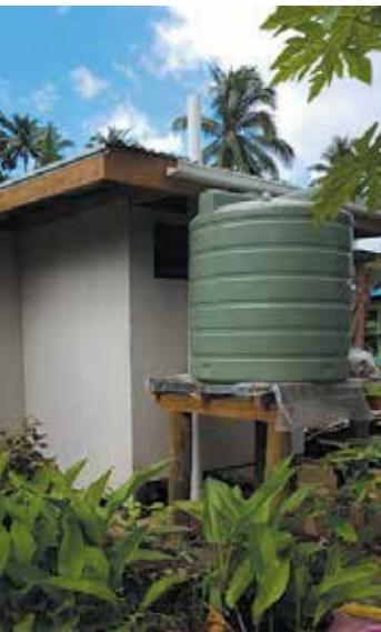
Above: Construction of toilet and shower units at Tamavua-i-Wai.
