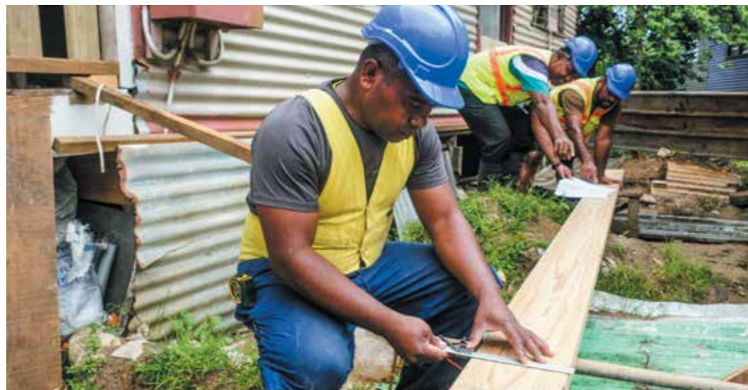
Paid community volunteers for construction are stimulating local pandemic recovery.
